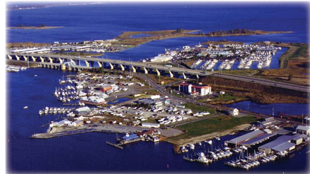
An aerial view of the Kent Narrows at U.S. Route 50/301
